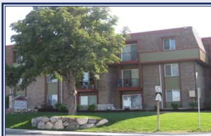
Time Square at the Brickyard 121 units - Salt Lake City, UT
