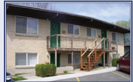
White Apartments 18 units - Salt Lake City, UT
